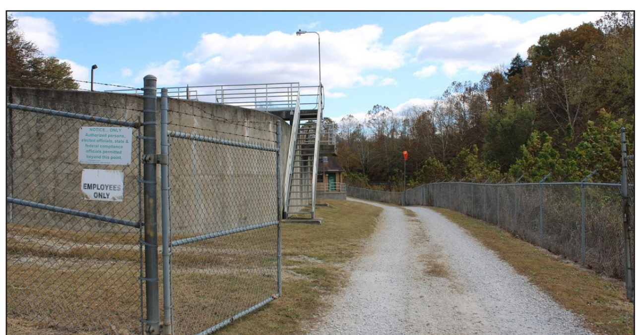
Olive Hill has struggled with waste water issues that a FIVCO grant could help alleviate with the assistance of their new engineering firm. (Photo by Jeremy D. Wells, Carter County Times)
