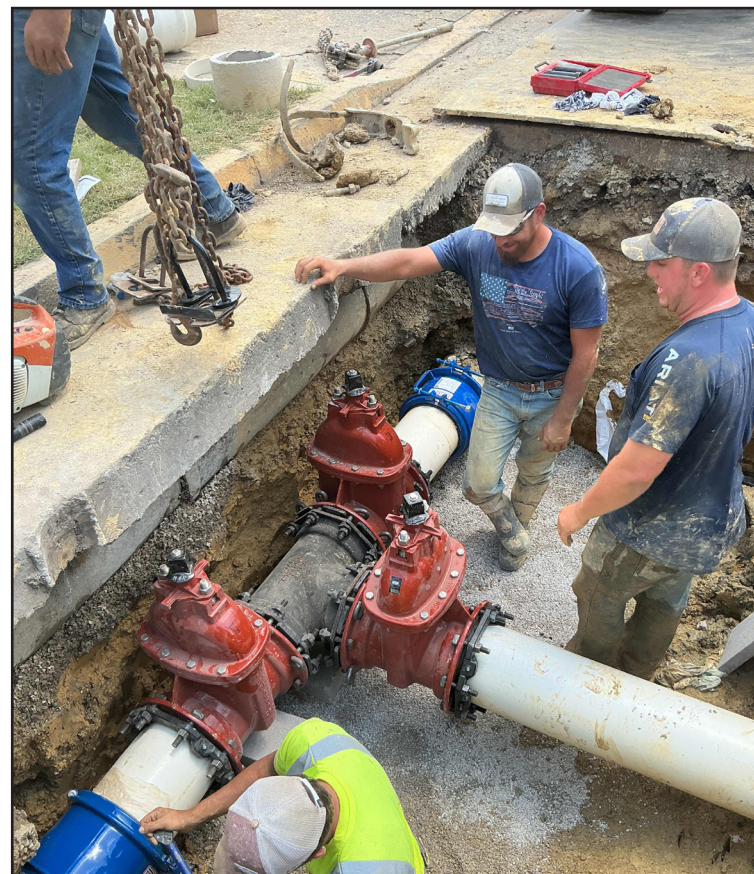
Utility crews work on replacing valves along Hord Street in Grayson. (Photo by Charles Romans, Carter County Times)
