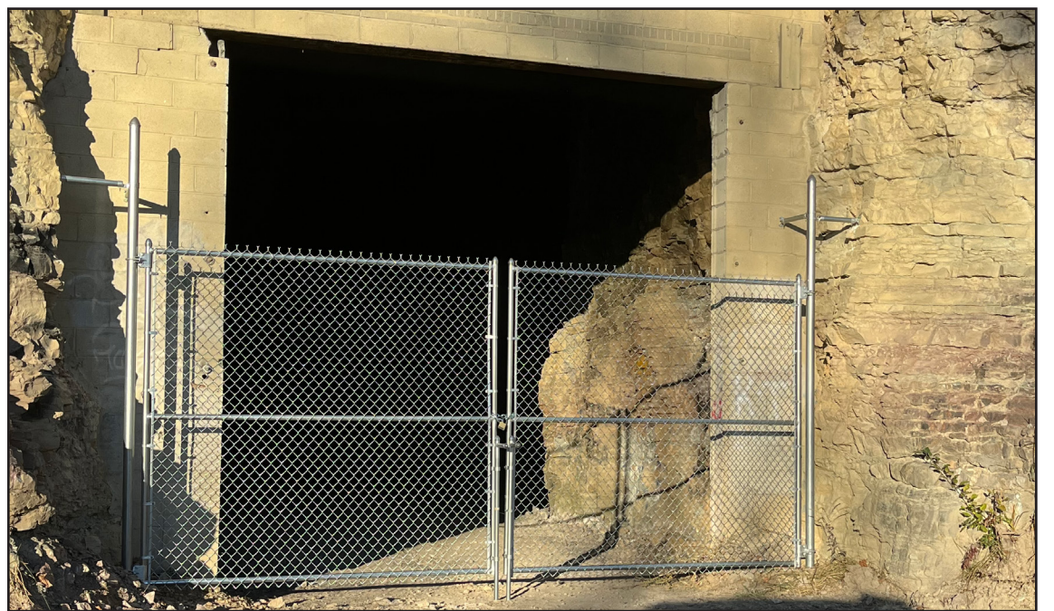
New fences surround the old Mushroom Mine as it's prepared for its new role as an underground training facility for mine safety. (Photo by Charles Romans, Carter County Times )
